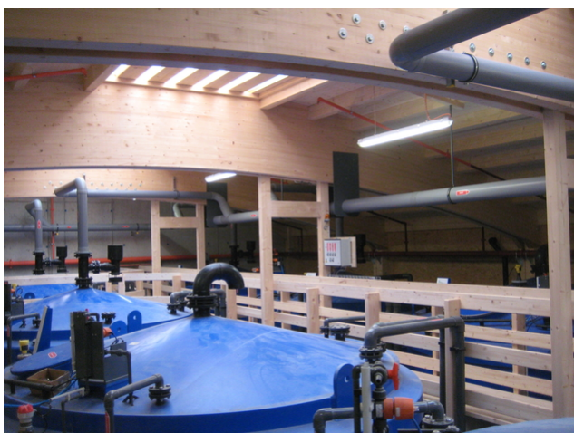
Hall de stockage zone 1
