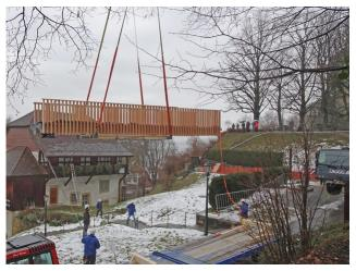
A crane lifted the 10.5 meter long bridge into place
