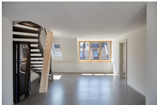
Visible brace in the apartment
