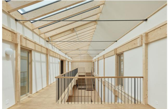
In the Generationenhaus Mooseggstrasse, a lot of beetle wood and almost no glued cross-sections are used. The skeleton construction is part of the architectural expression.
