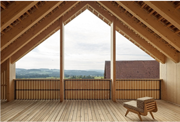
Roof cutout with a view of the Thurgau landscape
