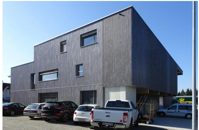
In Aefligen, between Bern and Solothurn, a commercial building with various ancillary rooms was built. The building with a volume of over 6,000 cubic meters convinces with its load-bearing structure and the facade made of wood.
