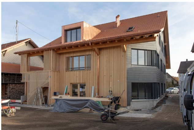
Fire protection facade to the neighboring house
