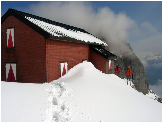
The original Dossen hut
