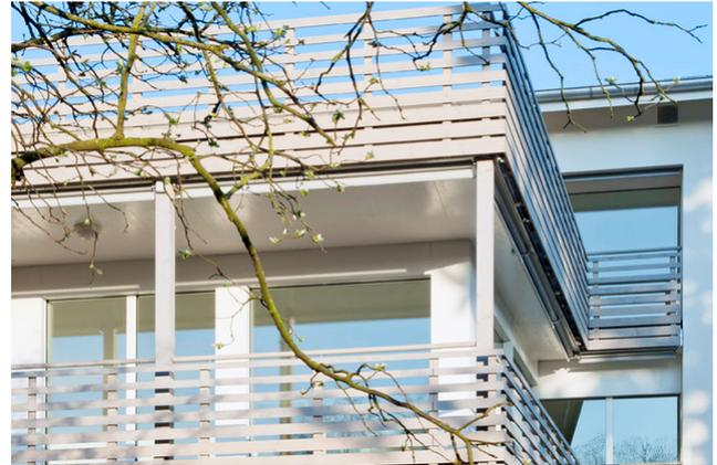
The existing apartment building on Salvatorstrasse underwent a total renovation to create more space, comfort and aesthetics. The living room extension consists of hollow box elements, which rests on a post and beam construction at the front and is clad with a glass front.
