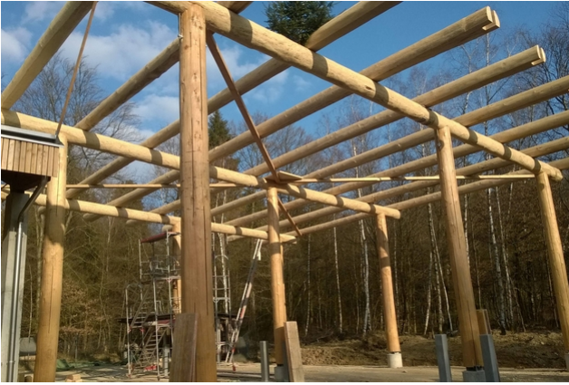
Supporting structure after assembly
