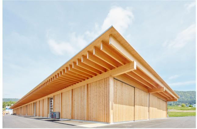
Cross-stacked supporting structure: the roof beams rest on the purlins
