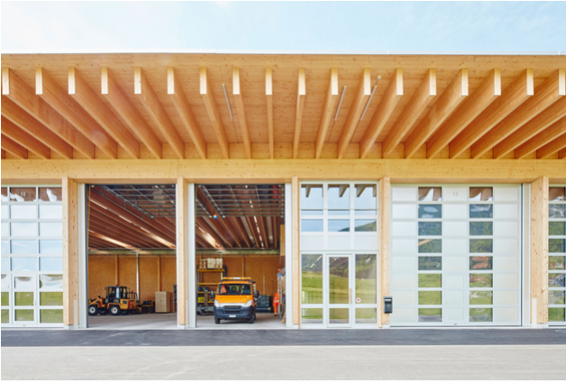
The work yard offers ample space for trucks, snow plows and other vehicles
