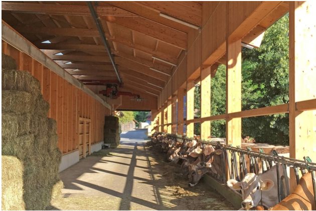
Interior view feed store
