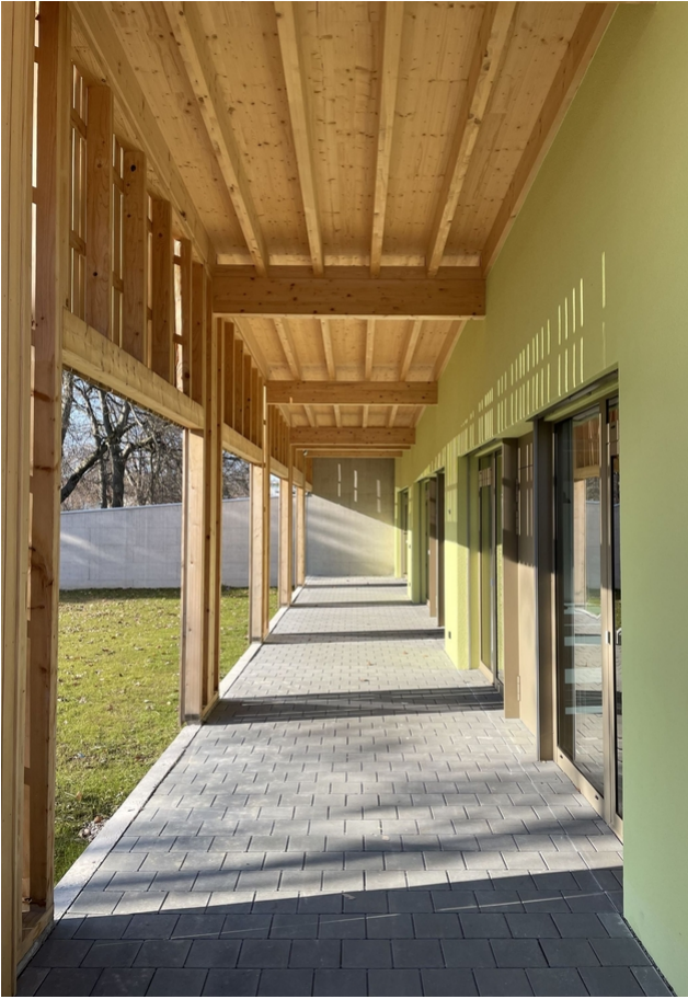
The portico with the visible joists
