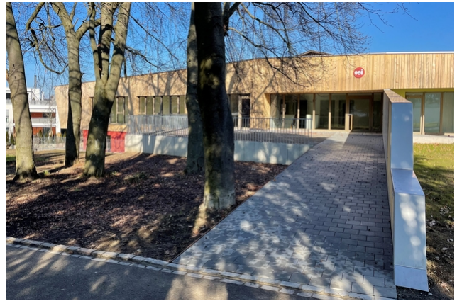
Construction and facade are made of wood
