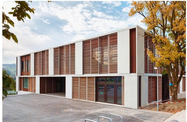
Wood characterizes the children's everyday school life at the Schachenmatten school building in Bonstetten. Built in 2015, the school building is a hybrid construction with concrete ceilings and load-bearing exterior walls made of wood. The example shows: Wood construction is also becoming increasingly important for public buildings.
