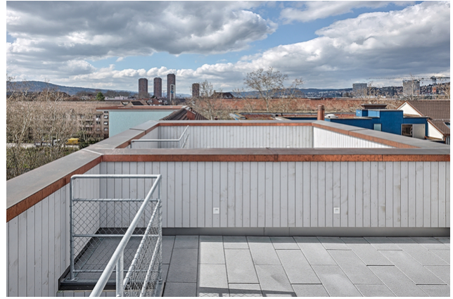
Roof terrace (Photos: Roger Frei Zurich)
