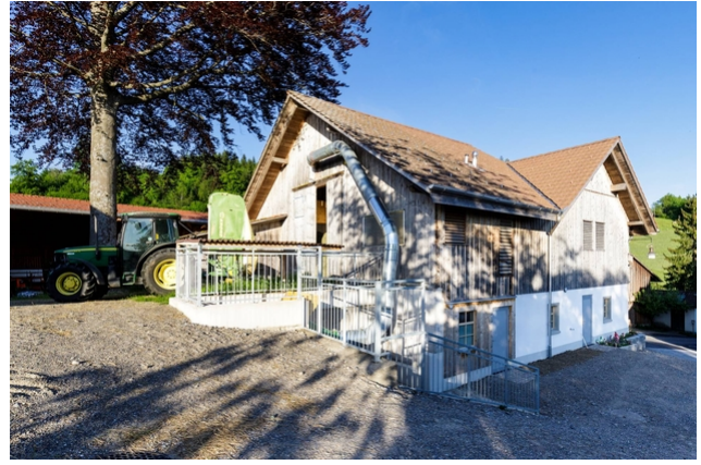
Exterior view of barn renovation
