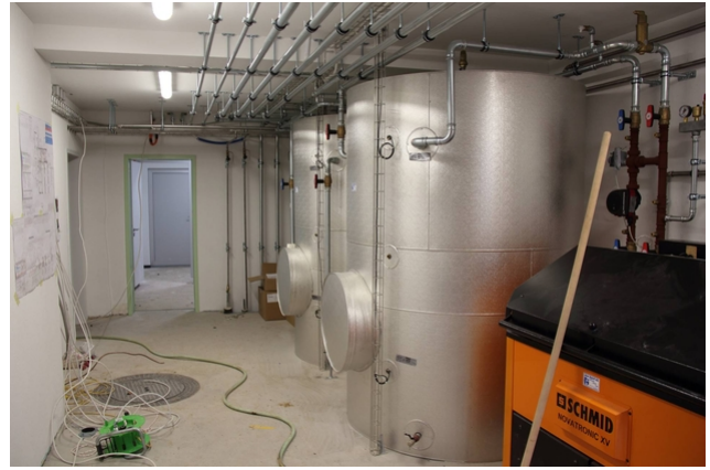
Building technology and building envelope are coordinated.
