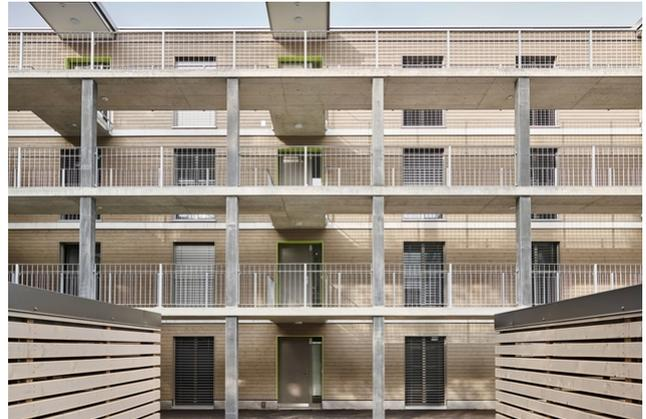
The new Brühlmatt apartment building, which was realized as a hybrid building, has 32 apartments in the middle of Urdorf. The apartments are accessible via open arcades that are slightly offset from the facade.
