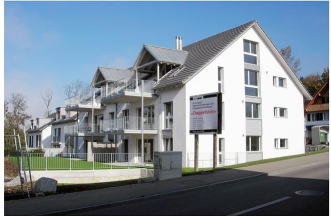
On the property on Zwillikerstrasse in Ottenbach, two MFAs were to be built. These comprise 2 and 3 floors respectively and contain 4 and 6 large condominiums. It is planned to build the walls, ceilings and the roof in optiholz® board piles. The walls outside will be insulated and plastered.
