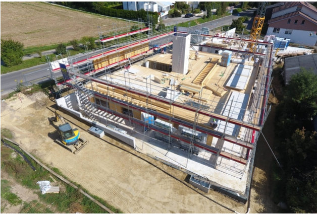
CLT lift shaft
