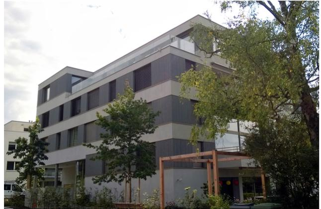
The MFH Ringstrasse is a replacement building in mixed construction with 14 apartments in Minergie-P-Eco standard and was designed according to the SIA efficiency path energy.
