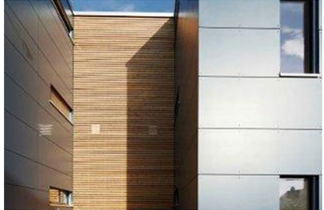
In a picturesque, elevated location on the south-western slope of Wohlen, this 6-family mini-house was realized in timber construction. The apartments are arranged as two-flats on both sides of the staircase and built in pure timber construction.
