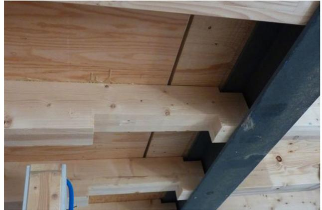
Cutouts for building services installations in the rib elements of the floor slabs
