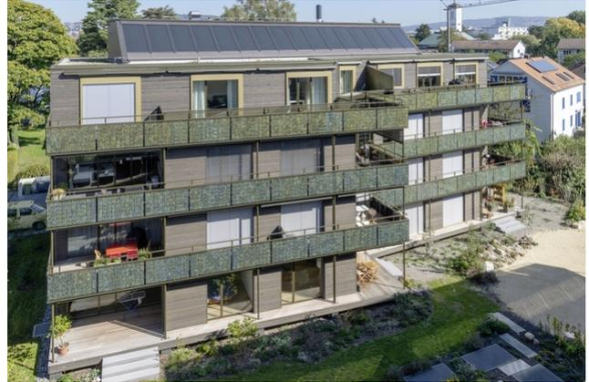
The new replacement buildings in Zurich Altstetten are among the first projects that can do without concrete in the stairwell as well. This has been possible since the revision of the fire protection guidelines in 2015.
