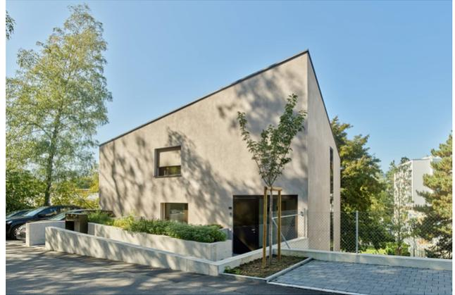
The apartment building in Kilchberg is completely built in wood, including staircase. The special feature: The wooden outer wall of the first floor is half buried in the ground.
