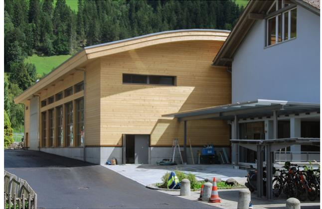
As a replacement for an old gymnasium, a modern multi-purpose hall was built in Lenk BE. The roof of the hall and its supporting structure are made of wood. The structure not only has to withstand high snow loads, but also the forces that arise when the sports equipment attached to the structure is used.
