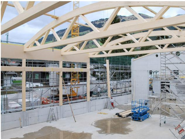
More supporting structure height due to the slightly upward curved bottom chord of the trusses
