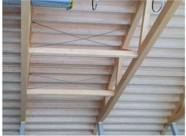
The stabilizing construction absorbs the forces of the sports equipment
