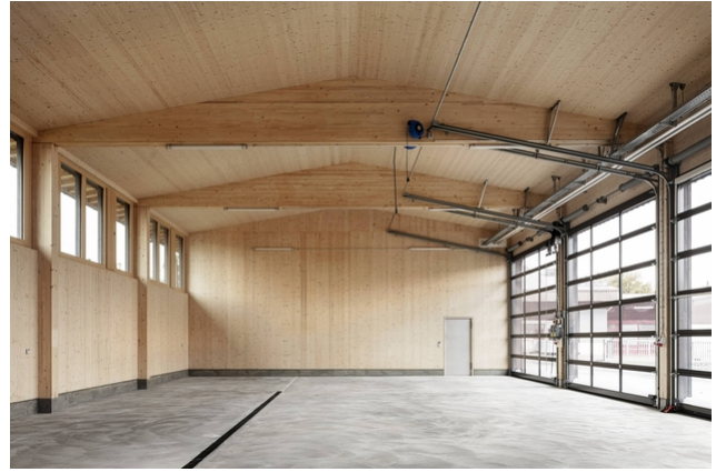
Large gates attached to the wooden structure (Lucas Peter, Zurich)
