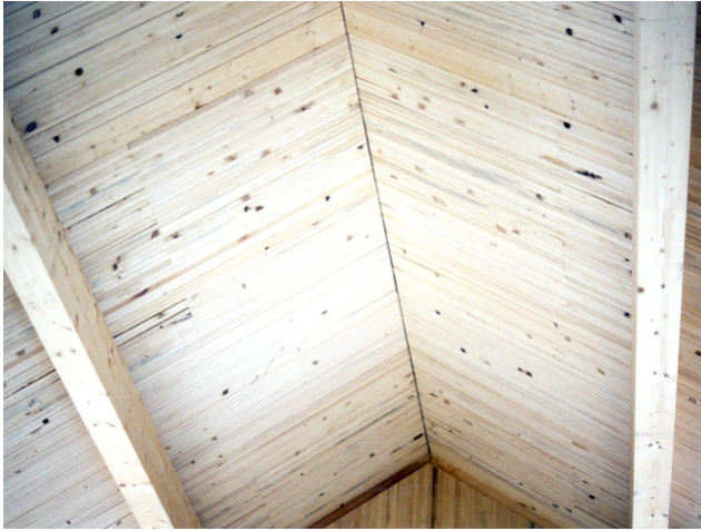
Roof construction with optiholz board stack modules
