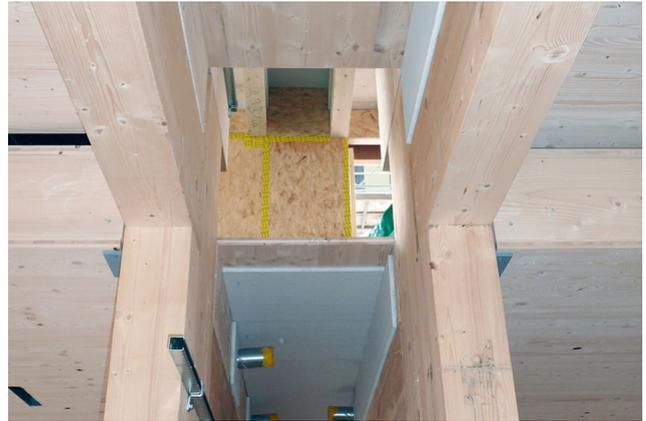
An exciting new building project on Habsburgstrasse in Zurich. A 5-storey MFH as a pure timber construction. Solid construction despite difficult fire protection conditions. The central staircase core and the fire wall to the neighboring building brace the column-slab construction.
