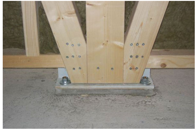
Anchoring earthquake bracing
