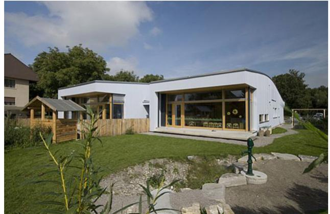
The new double kindergarten in Uttigen was planned and executed as a pure timber construction. The building should have a simple and inexpensive construction. The use should also remain variable - school meetings should also be able to take place there.
