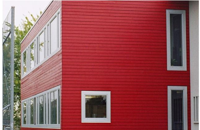
Here, a two-story rucksack addition to the existing building was to be realized, with adaptation of the existing eaves and transitions to the first building. The facade was to be created with a painted wooden formwork.
