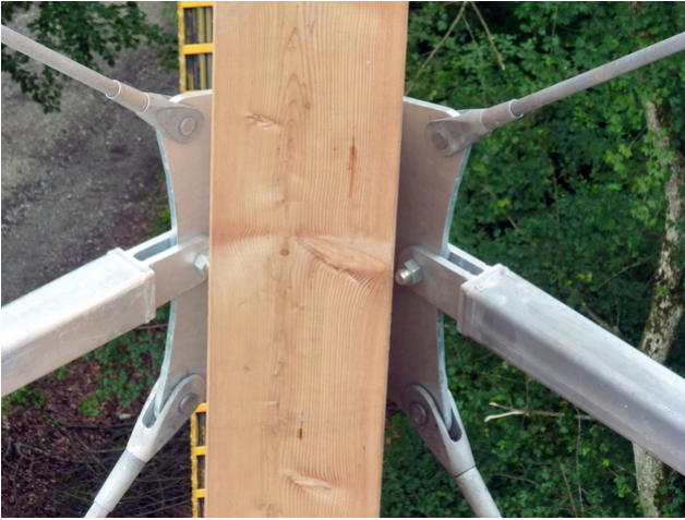
Tension and compression rod connection
