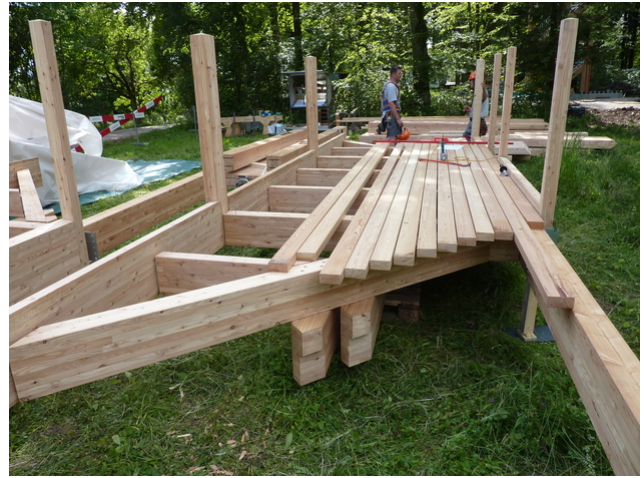
Assembling the tower
