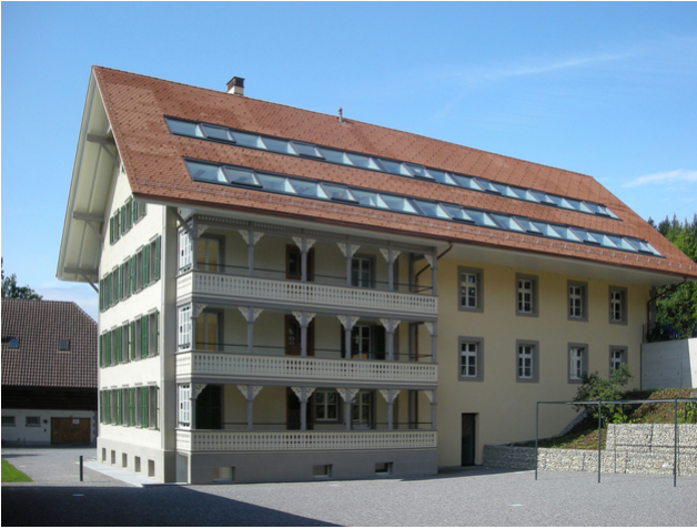
Mill building renovated
