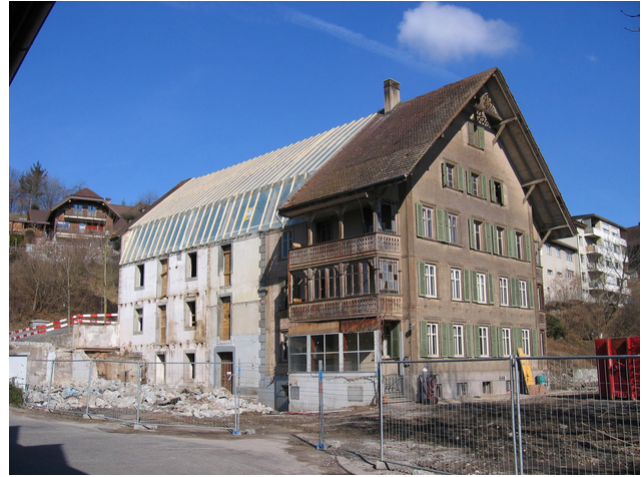
Mill before renovation
