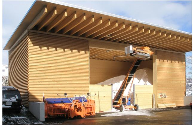
Due to damage to the concrete and steel structure, the existing salt storage hall at the road inspectorate's depot in Seftigen had to be replaced.
