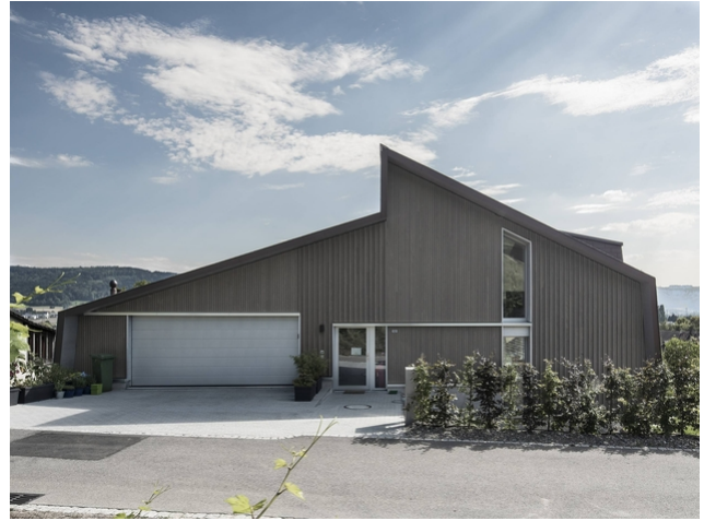
The garage directly above the bedroom made high demands on sound insulation
