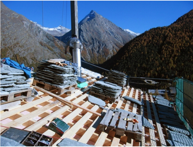
Roofing with natural stone slabs
