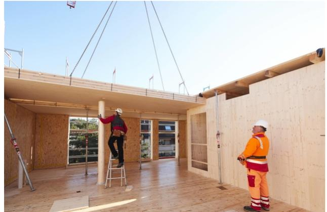
In Frenkendorf, the first four-story column-and-slab structure made of wood was built. Thanks to TS3, the building once planned in concrete can be built in wood. The planning with the multi-axial load-bearing cross laminated timber panels is similar to reinforced concrete.
