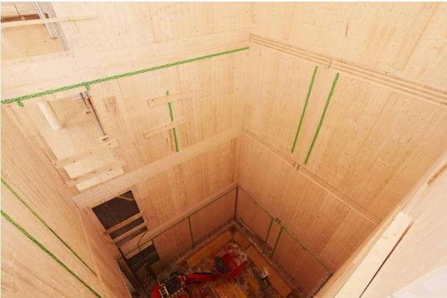
The staircase core is in place. The liquid concrete is poured in afterwards
