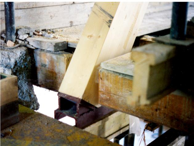
UNP beam, end support truss
