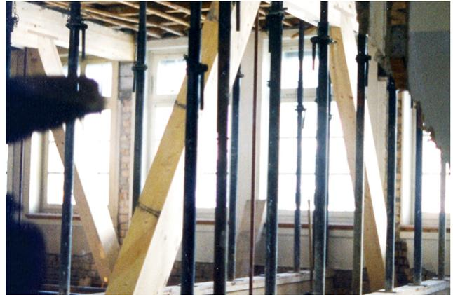
The existing building in the center of Thun was converted into business premises and apartments. On the 1st floor, three high reinforced concrete girders were installed, which protruded from above about 70 cm into the clearance gauge. The planned store was to be column-free with a smooth soffit. The existing beam layers were to remain unchanged.
