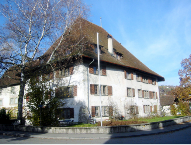
Exterior before renovation
