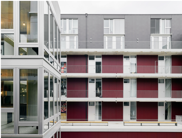
The apartments of the MIN MAX development are accessible via arcades
