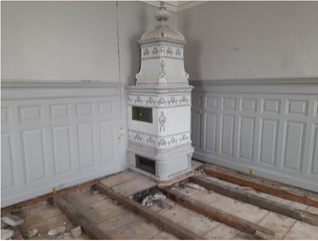
Floor slab before retrofitting
