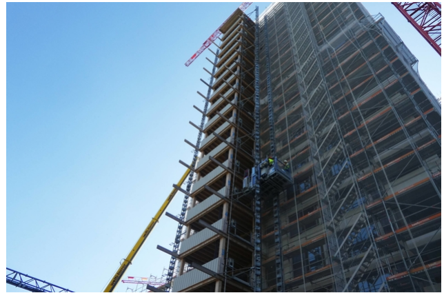
Scaffolding tower from below
