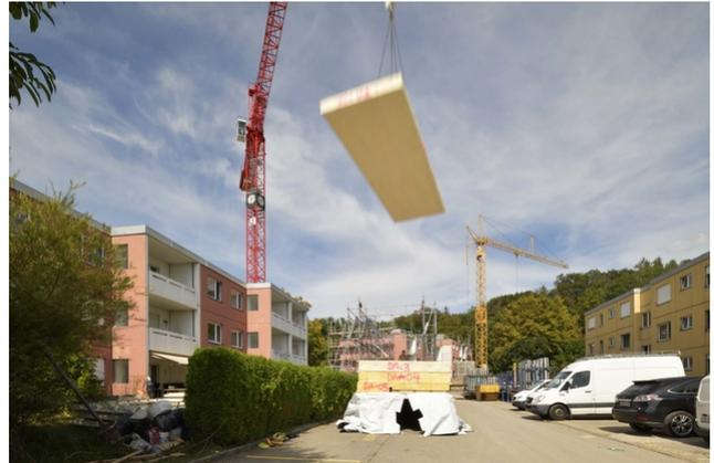
In the middle of the city of Wetzikon in the canton of Zurich, a housing estate was renovated. By adding wooden floors, 36 new residential units were created on top of the prefabricated buildings designed by the architectural icon Ernst Göhner.
