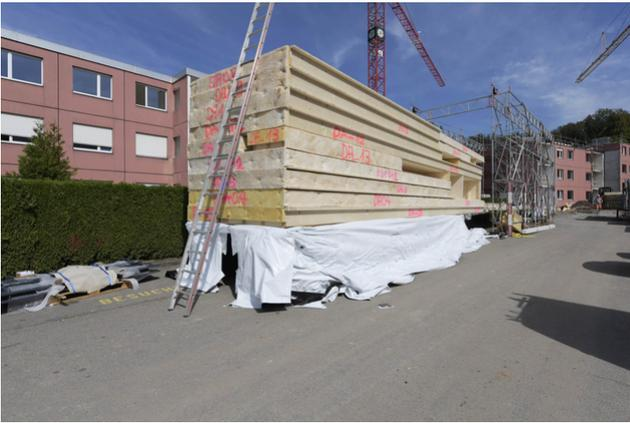
Delivery of the prefabricated wooden elements
