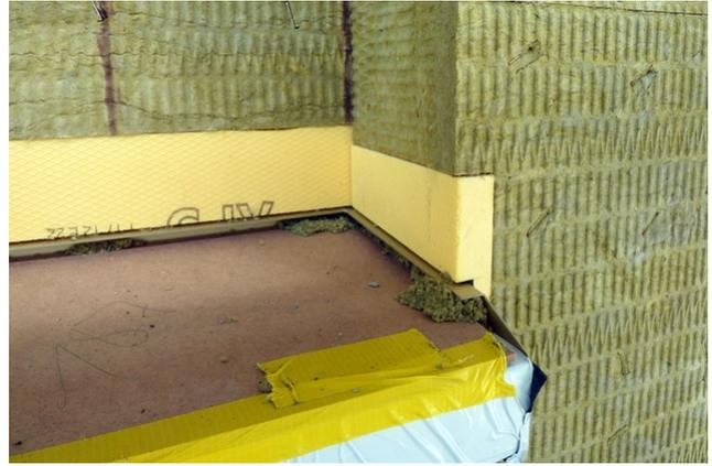
Detail insulation on window sill
